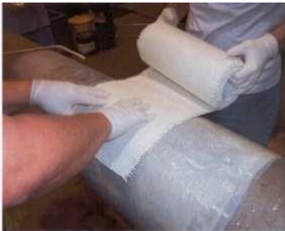
Figure 6 - First layer of Aqua Wrap installed on pipe
