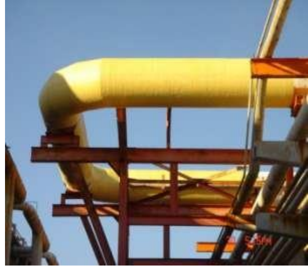
Salina Cruz Refinery, Mexico, 60 inches line (150cm) at 350 psi (24.2 Bar).
