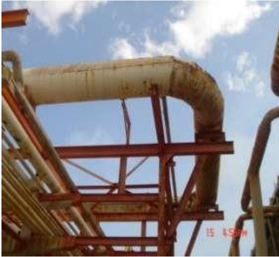
Salina Cruz Refinery, Mexico, 60 inches line (150cm) at 350 psi (24.2 Bar).
