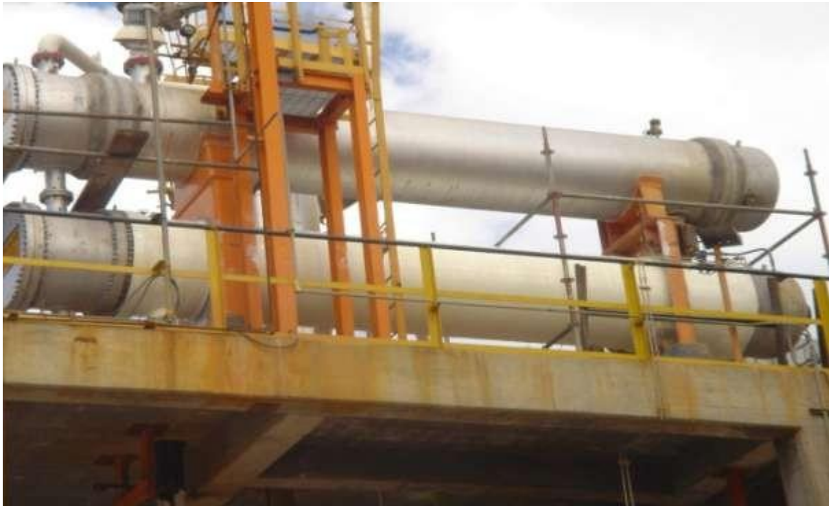
Salamanca refinery. Heat exchanger, 250°F (121°C) at 250 psi (17.2 bar).
